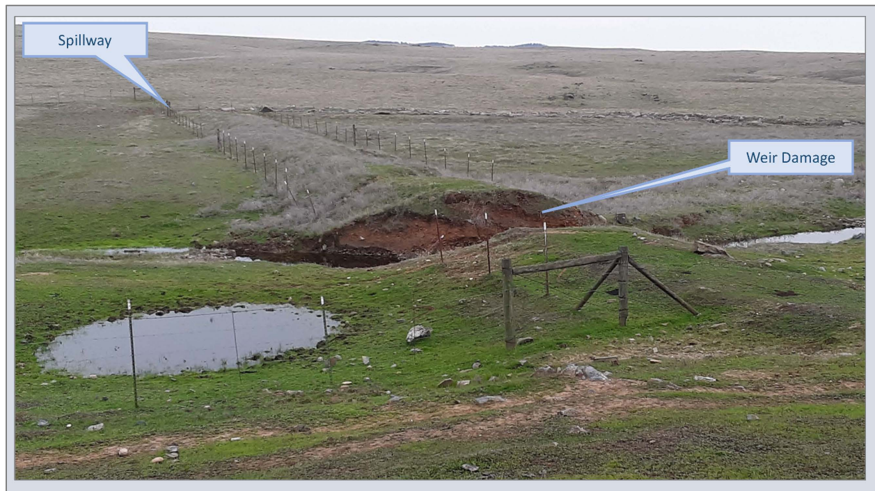
Figure 4. Erosion compromised impoundment #2, looking west, with VP#8813 in foreground, within the Blackbird Basins Action Area
