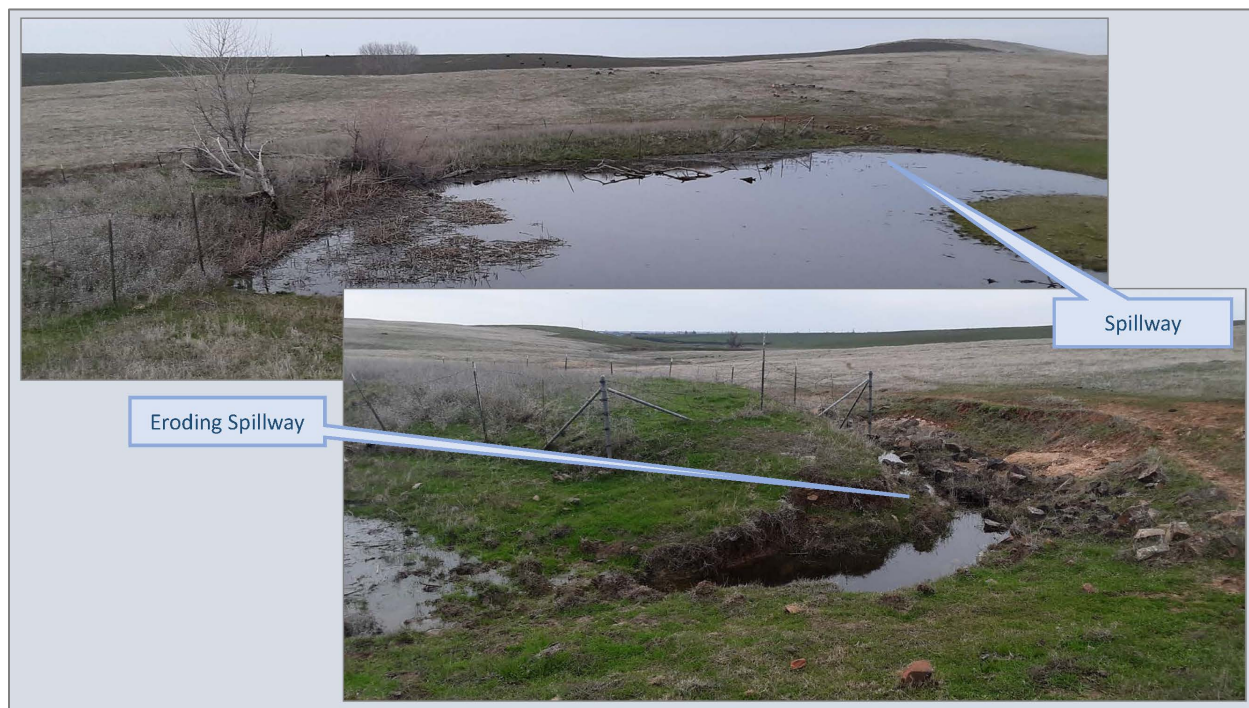
Figure 6. Current condition of impoundment #4 (above) and the eroding spillway (below), looking north, within the Blackbird Basins Action Area
