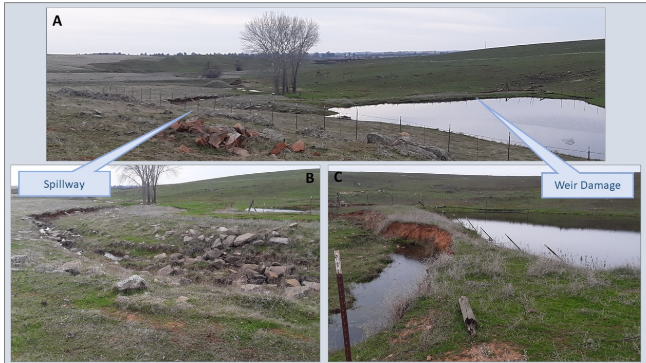
Figure 3. Impoundment #1 (A), incised spillway looking SW, (B) and downstream erosion looking SW, (C), damaged impoundment looking west, within the Blackbird Basins Action Area
